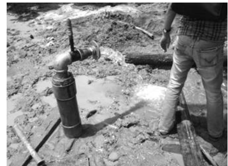
Fig.2 Flowing artesian well in Mae Sai basin, depth of 200 meters with 50-60 m 3 /hour.
