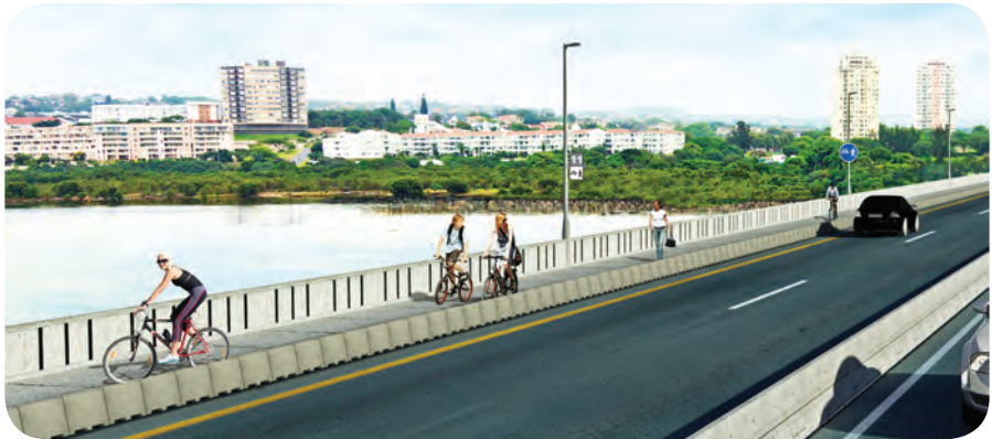
▲ The bridge across the uMgeni Estuary has been widened to accommodate cyclists
