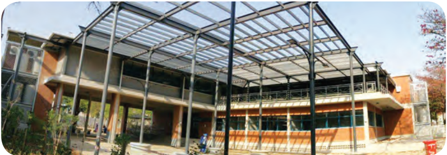
▲ The eThekwini Water & Sanitation Customer Centre has an energy and water efficient design.
