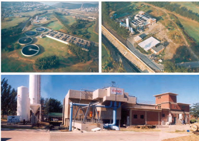
▲ Southern Wastewater Treatment Works
