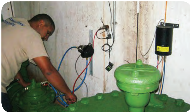
▲ The i20 pressure sensor helps reduce water loss in the municipality
