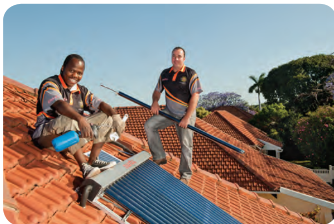
▲ Installing solar water heaters in the Shisa Solar Programme
