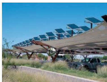
► Figure 3: PHOTOVOLTAIC PANELS CREATE COVERED PARKING FOR VISITORS AND GENERATE ENOUGH SOLAR ENERGY TO POWER APPROXIMATELY 70 PERCENT OF THE SPRINGS PRESERVE
