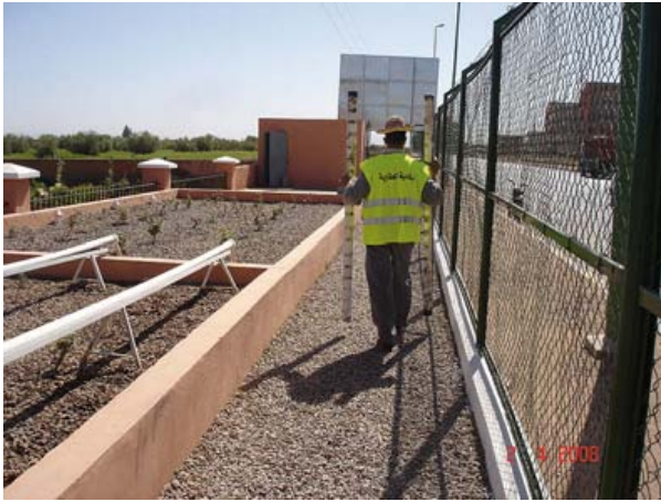
▲ Figure 6: MUNICIPALITY WORKER IN DUTY IN THE GW TREATMENT PLANT
