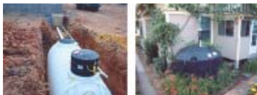
Fig. 2: UNDERGROUND AND ABOVE- GROUND CISTERNS
