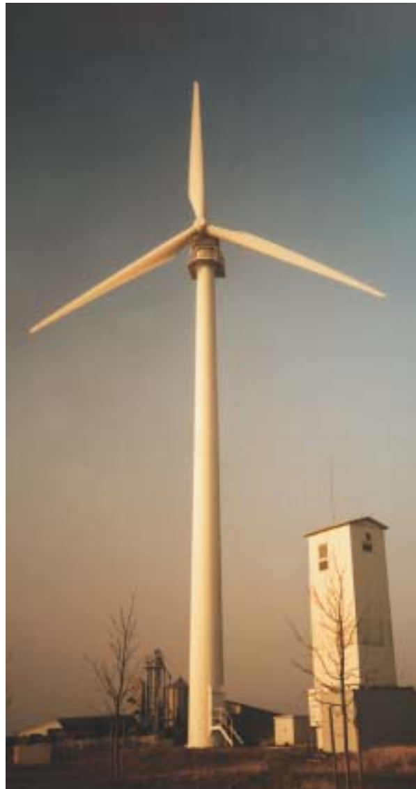
Fig. 4: OUTSIDE VIEW OF THE WIND DRIVEN DESALINATION PLANT
