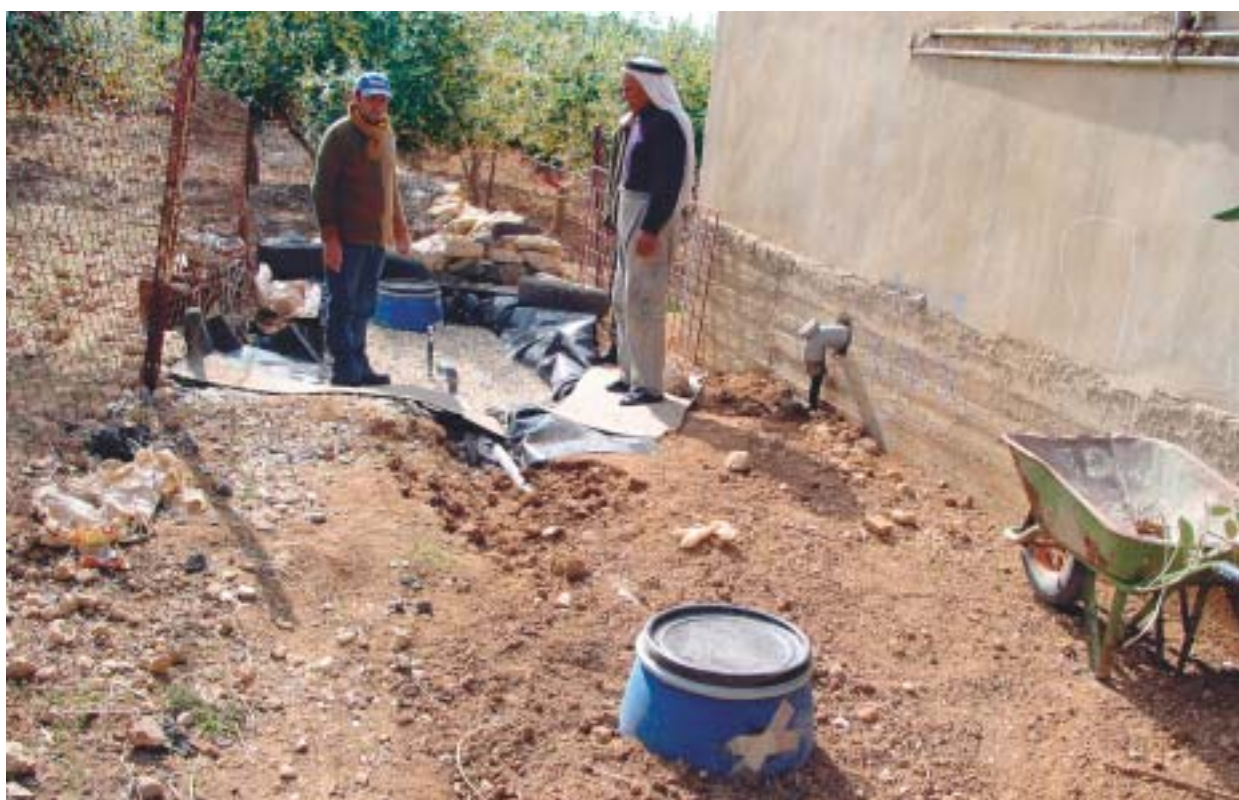
Fig. 3: CONFINED TRENCH SYSTEM
