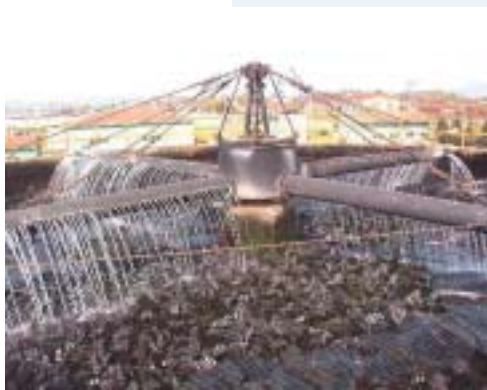
Fig. 2: TRICKLING FILTER WITH ROTATING SPRINKLER
