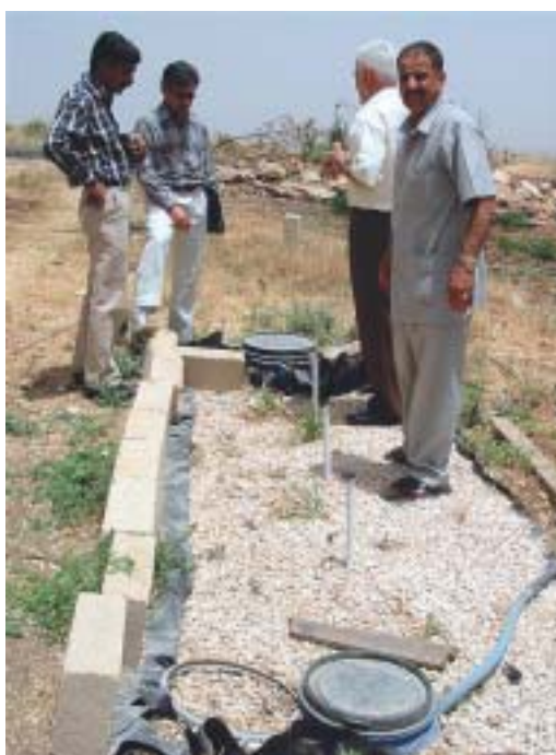
Fig. 2: INSTALLED CONFINED TRENCH GREYWATER TREATMENT SYSTEM
