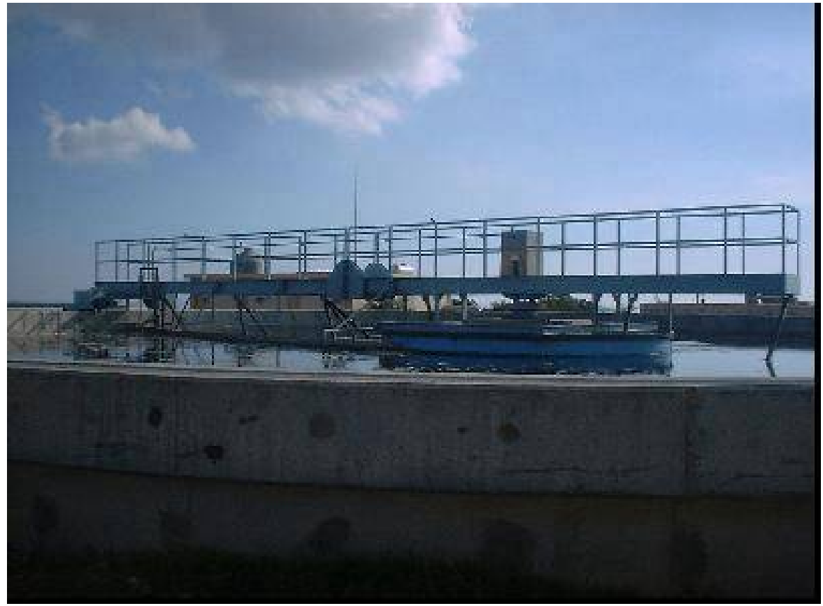
Figure 13. Settlement Tank.
