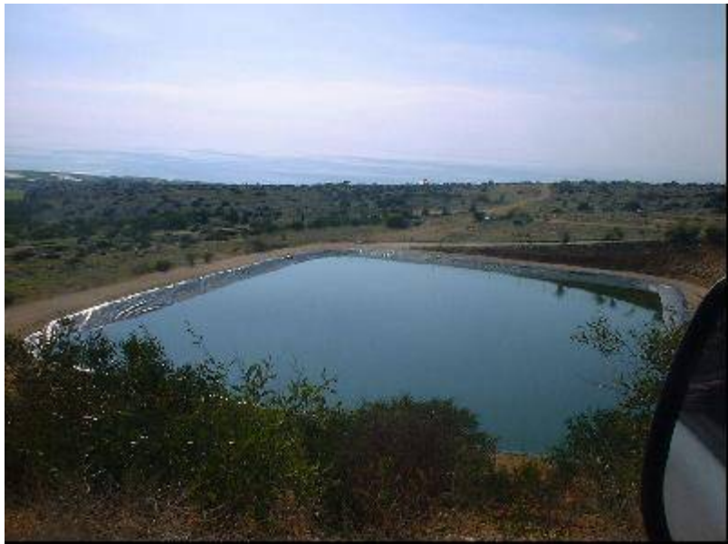
Figure 15. Storage Tank (Secondary treated water).
