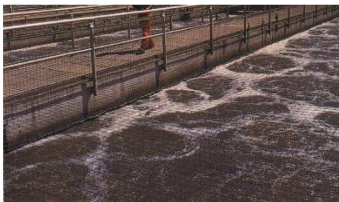
Figure 53. Pre-aeration tanks.
