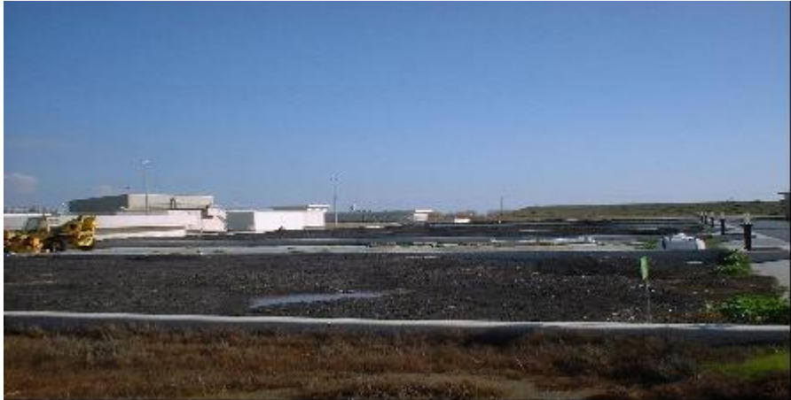
Figure 10. Sludge Drying Beds.
