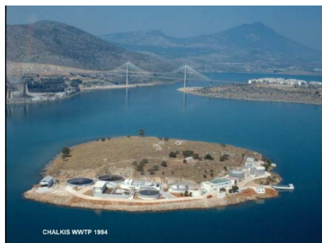
Figure 17. Advanced Wastewater Treatment for Reuse at the WWTP of Chalkis.
