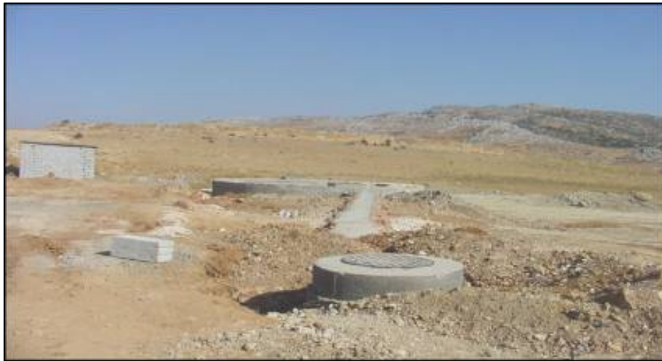
Figure 30. The Yanta Plant facing power supply problems.
