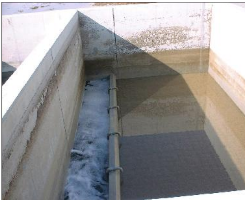
Figure 7. Sand Filter.
