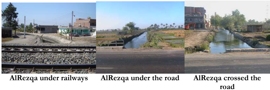
Figure 20. AlRezqa canal crossing the railway and agricultural road at Mostapha Agha Village now
