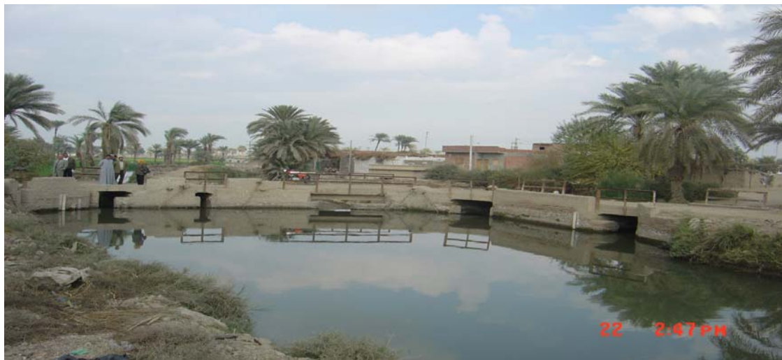
Figure 14. Gates of the Seila canal to the distributary canals
