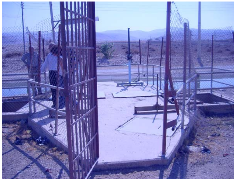
Site Visit – July 2007 – Turn Out
