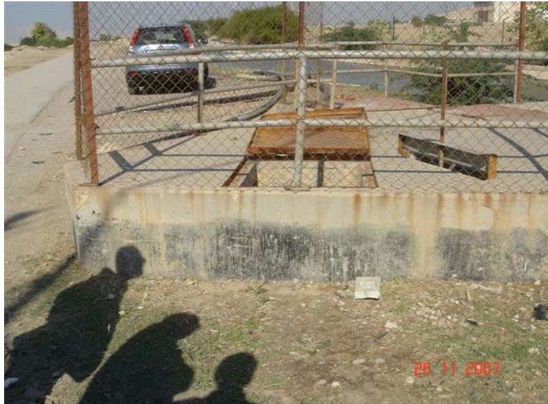
Site visit – November 2007 – Turn Out 95 (G25)
