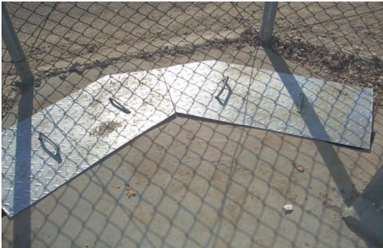
Turn Out 95 (p25) – Detail mainhole inspection King Abdulla Canal – Jordan – August 2008
