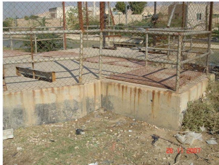
Site visit – November 2007 – Turn Out 95 (G25)
