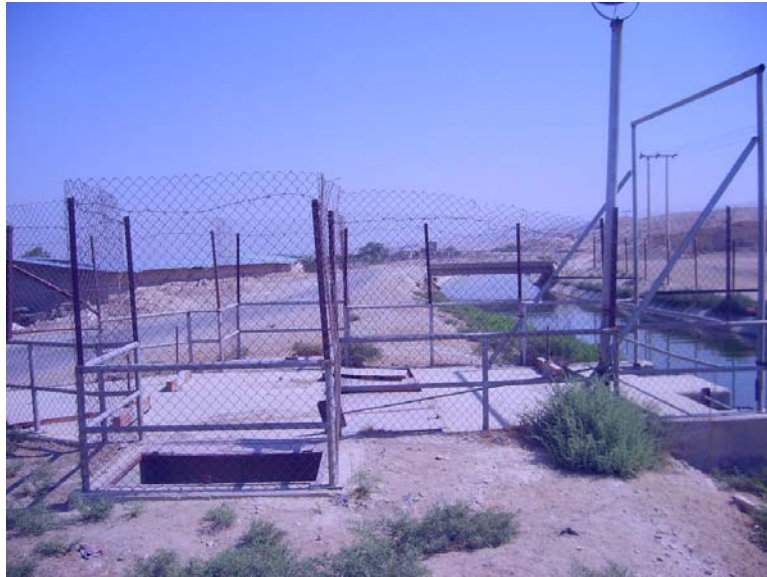
Site Visit – July 2007 – Turn Out 91 (p21)
