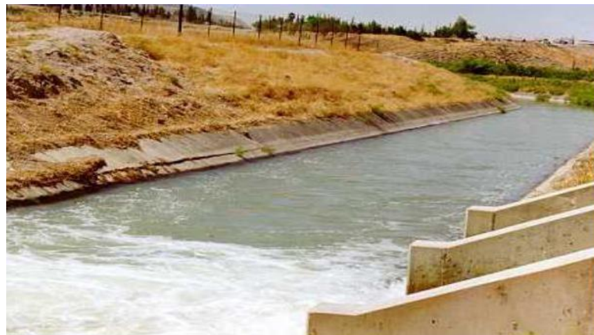
View of the KAC in northern Jordan Valley area
