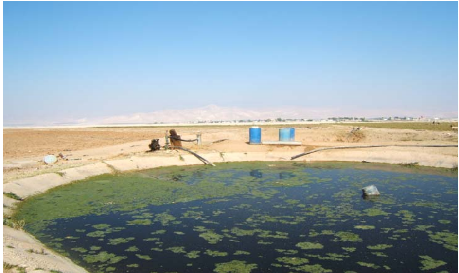
Common on farm pond, often invaded by algae. In this case, an old under-sized screen filter is placed between the diesel pump and the irrigation net.
