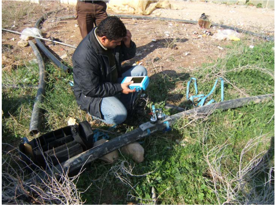
Checking the flow on the mainline by the portable ultrasonic clamp flowmeter
